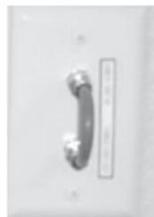
1. Remove the jumper wire from the coax faceplate.
