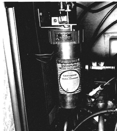
Fig. 4—Water Pump and Filter
